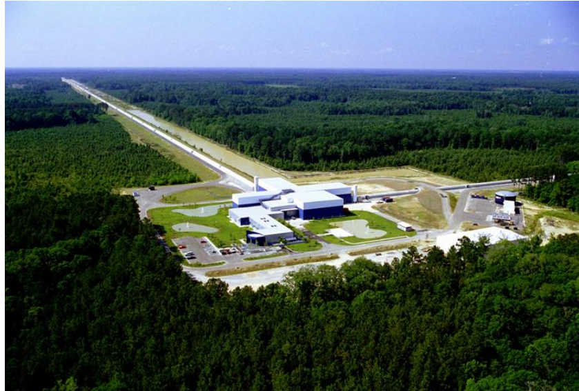
Laser Interferometer Gravitational-wave Observatory in Livingston, Louisiana. Each of the two arms is 4 kilometers long. LIGO has another such observatory in Hanford, Washington.
